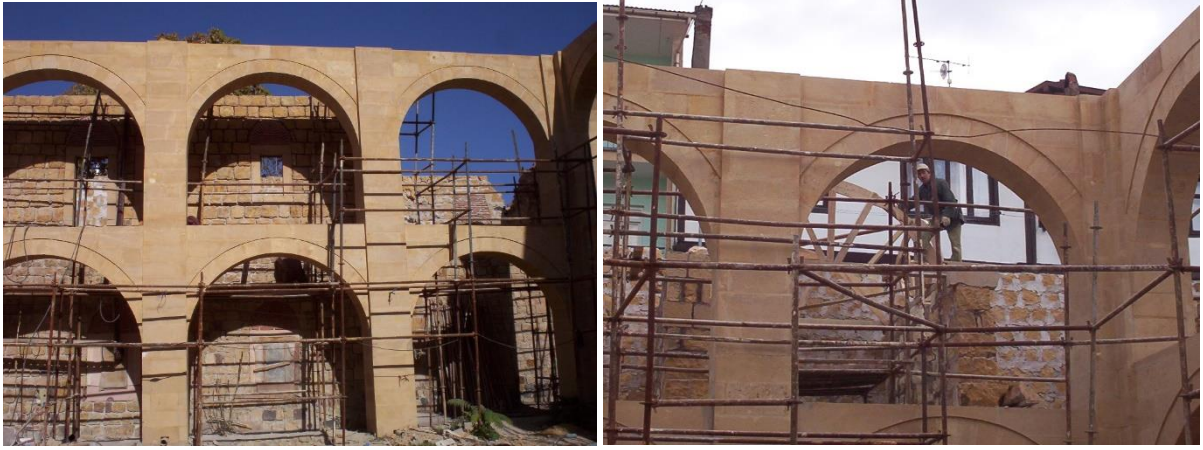
Figure 9. Cut stone arch manufacturing
