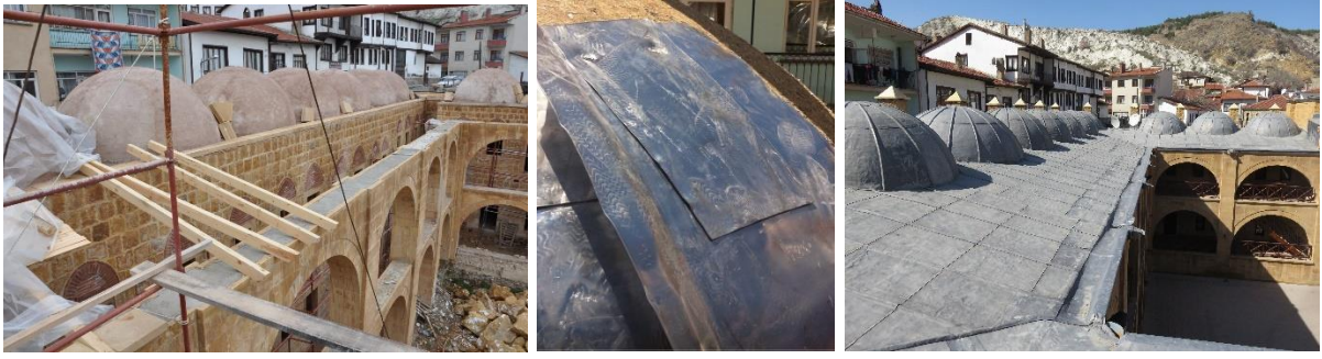
Figure 16. Mud plaster and lead productions in the dome
