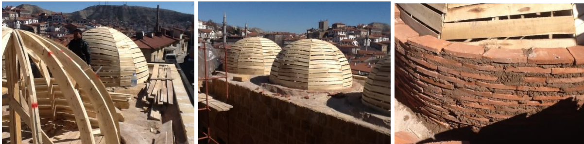
Figure 15. Dome manufacturing on the upper cover
