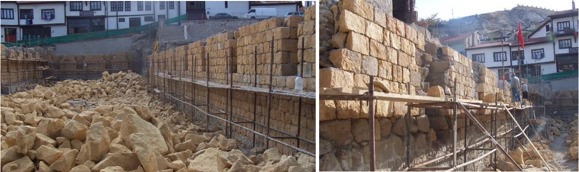
Figure 11. Rubble stone wall manufacturing in the shelter section
