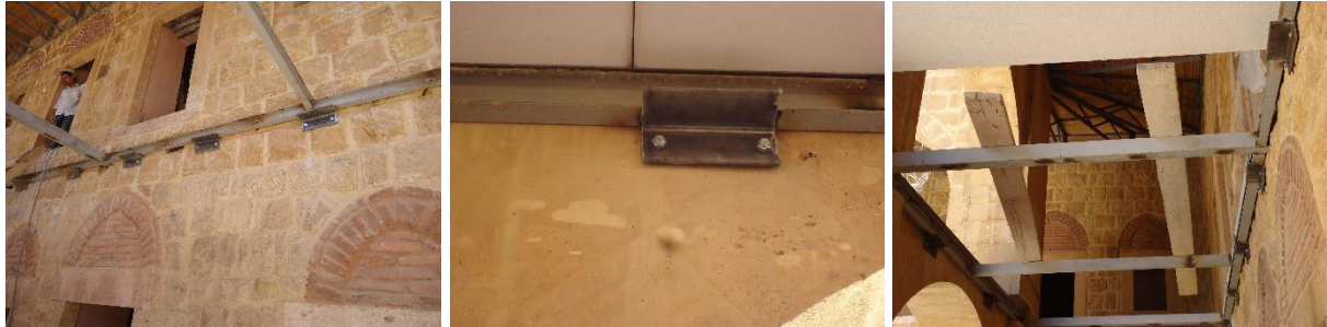
Figure 14. Steel and aerated concrete applications in the portico
