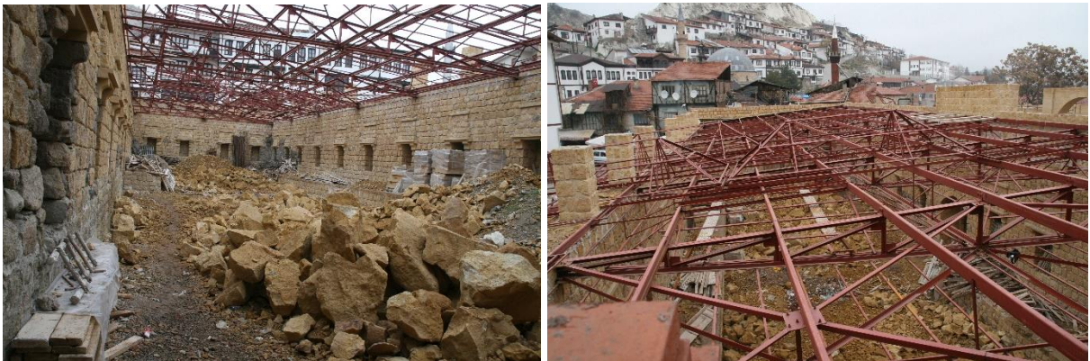
Figure 12. Shelter (develik) section steel roof manufacturing
